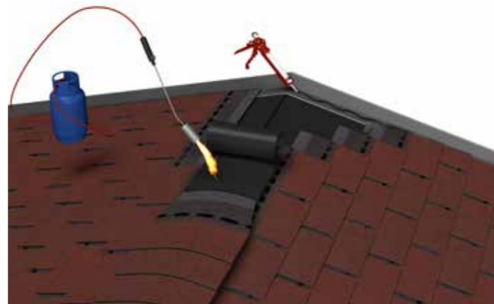
Hip and ridge on concrete deck by torch-on method
